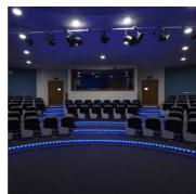
Gradus step lighting profiles use a modular design which makes maintenance and refurbishment work easy. The step profiles were installed with full cable management to hide all wires, creating a neat finish and preventing trip hazards.
